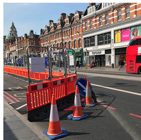
Figure 31: Footway widening outside station entrance – London
