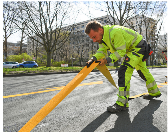
Figure 28: Pop up cycle lanes being installed. – Berlin (Copyright, Reuters images)
