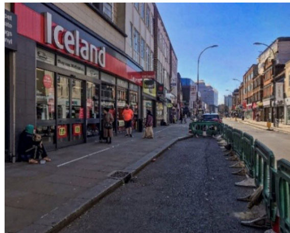
Figure 7: Widening of footways to accommodate queuing outside Iceland supermarket – London
