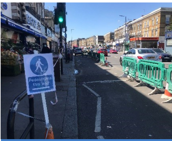
Figure 8: Physical barriers to separate vehicular traffic and widen pedestrian space – London
