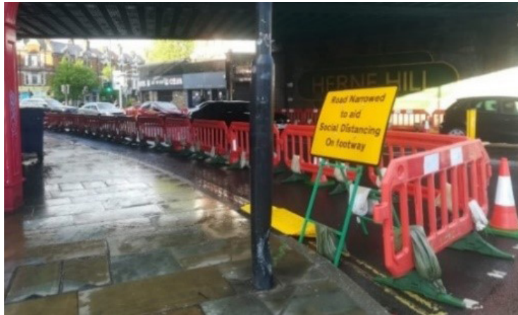
Figure 11: Physical barriers to separate vehicular traffic and widen pedestrian space – London
